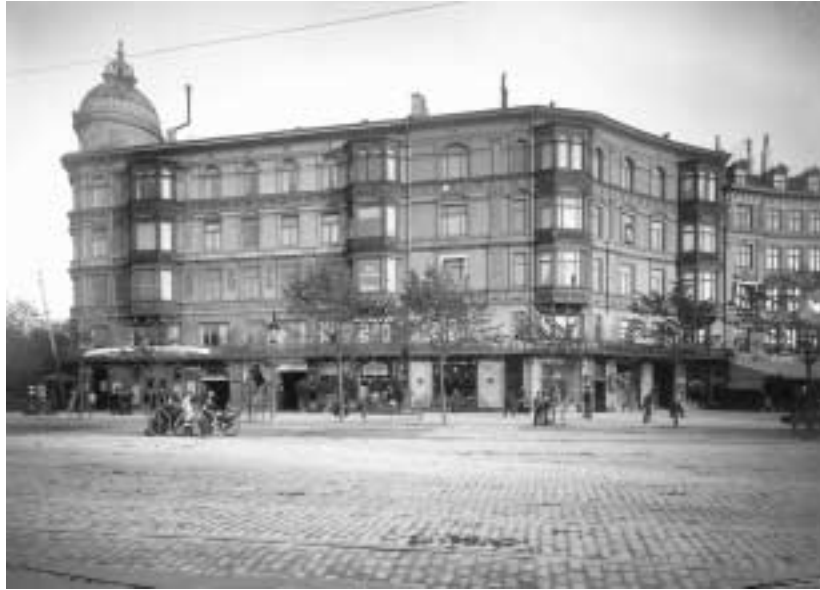
FIGURE 1.4. Exterior photograph of the Panoptikon building, located at Vesterbrogade 3 in Copenhagen, ca. 1903. The entrance to the Panoptikon is to the left; a sign advertising the Danish Folk Museum is visible in the second-floor window. Photo courtesy of the Royal Library (Copenhagen).
