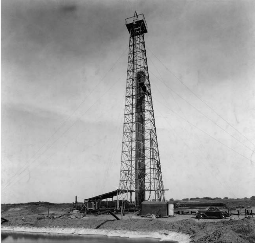
This 1940s rig could drill through to the bottom of the oil window. Derricks like this, although rarely used after 1950, are still a visual metaphor for the oil industry. © Bettmann/CORBIS.
